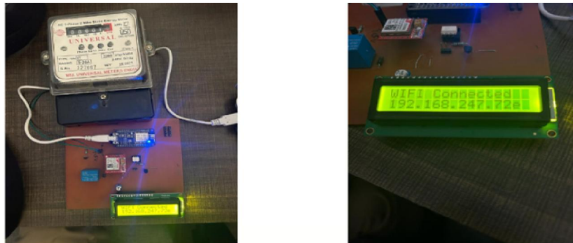
Fig 3. Energy Meter and LCD Display
