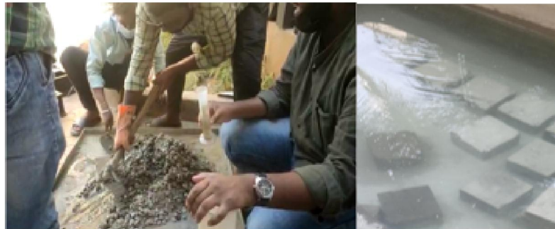
Fig 4: Preparation of Concrete
