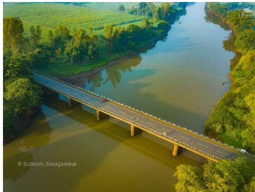
Fig no. 02 Bhadagaon bridge
