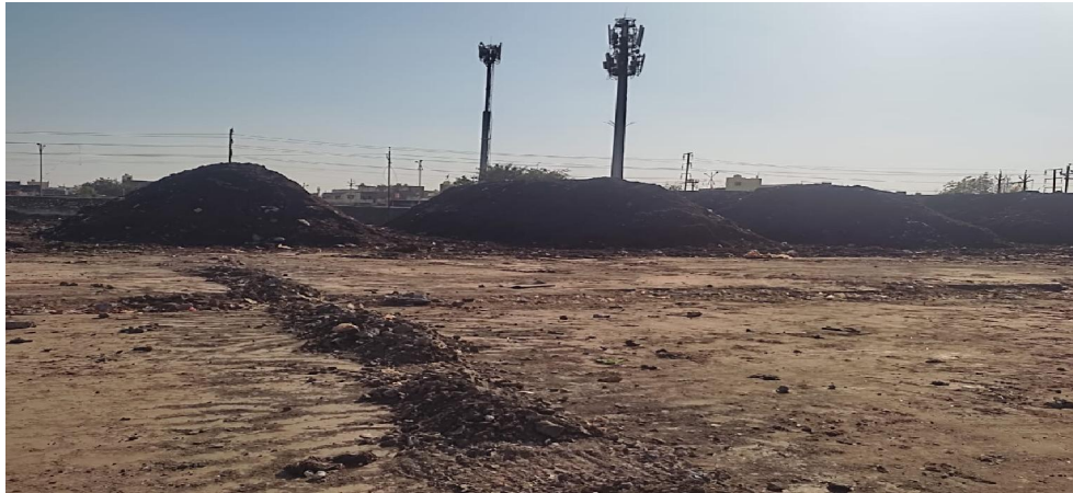
Bhandewadi Municipal Solid Waste Treatment Plant, Nagpur
