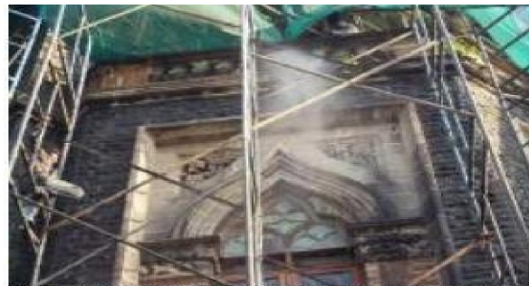
Using misting technique to remove years of dirt, dust and pollution.
