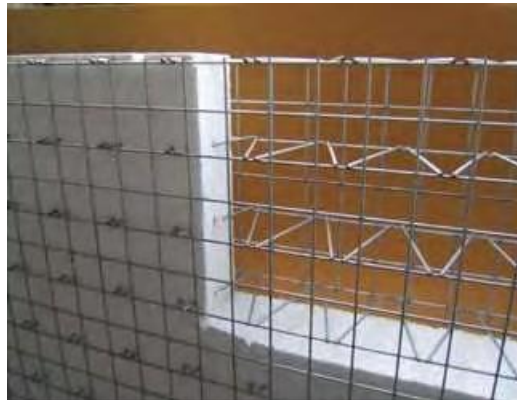
Fig 8.6- Reinforcing mesh expanded polystyrene core and diagonal wire.
