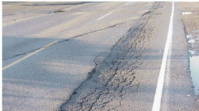
Figure 3: Rutting example
