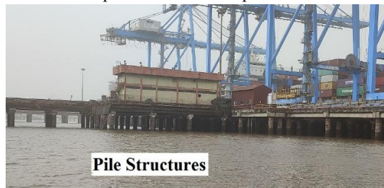
Fig 1.1 A Typical Pile Structure
