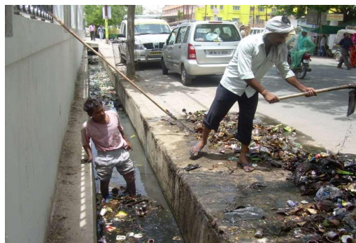
Figure 1: Manual Cleaning Of Drainage
