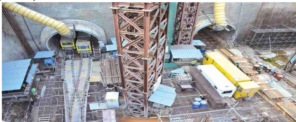
Figure 3.1: Underground metro construction work
