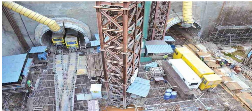
Figure 3.1: Underground metro construction work
