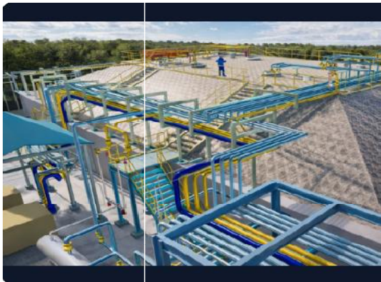
Figure 5.3 Mounded Storage Vessel
