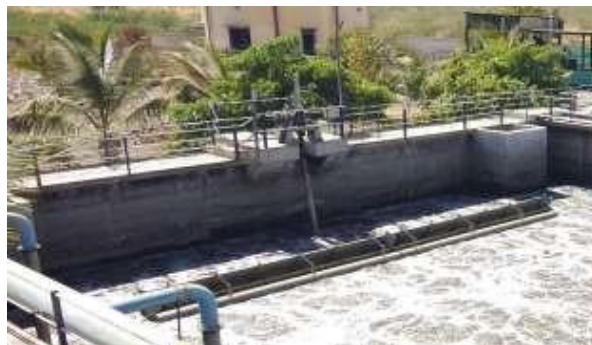
Fig 14: Decanting Unit
