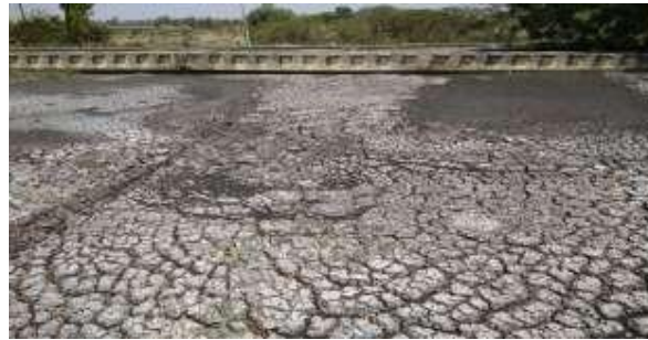
Fig 8: Sludge Drying Beds
