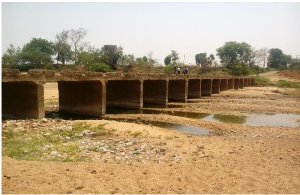
Figure 3: Multi Cell Box Culvert
