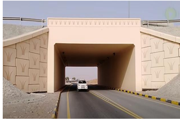
Figure 4: Vehicular Under Pass
