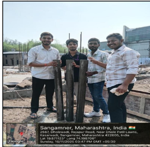
Fig.7. Concrete Filling Procedure
