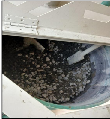
Fig 4: Concrete Mixing Process
