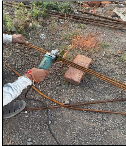
Fig 6: Rebar Cutting
