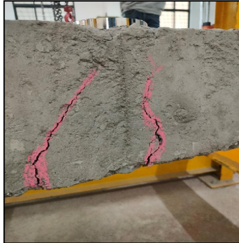
Fig 13: Multiple Crack Formation in Concrete Beam
