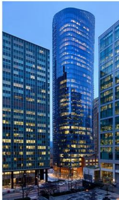
Figure 1: MNP Tower in Vancouver BC
