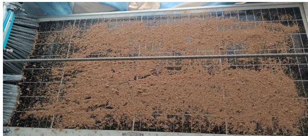
FIGURE VIII SOLAR PANEL COVERED BY DUST AT 90%
