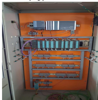
Fig. 2. Distributed Control System (PCS7) module with Input Output Racks
