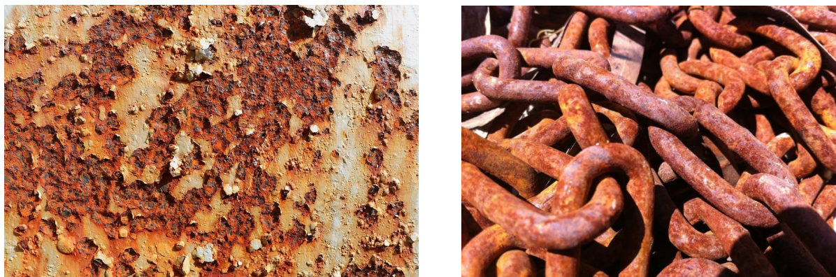
Figure 1: Corrosion of Iron Metals
