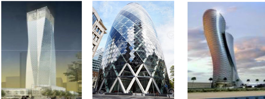
Figure 1: Diagrid buildings: (a) Jinling Tower in china, (b) Swiss Re in London and (c) Capital Gate Tower in Abu Dhabi
