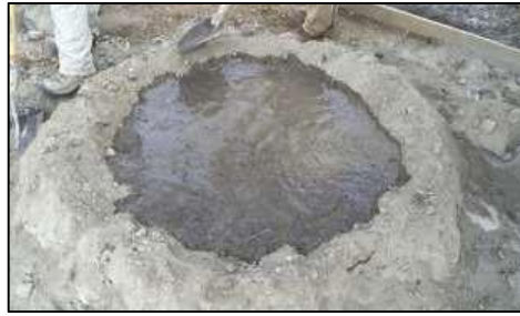
Figure 2: Hand Mixing of Concrete
