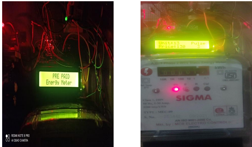
Figure 4: Working smart energy meter when no theft has occurred
