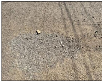
Fig- 12: Filled Pothole with HDPE Plate
