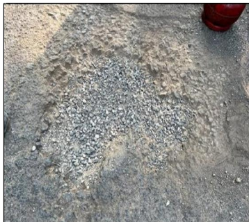
Fig- 8: Pothole Covered with Aggregate
