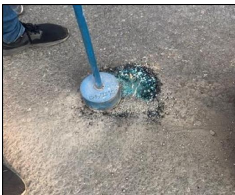
Fig- 11: Compaction with Rammer
