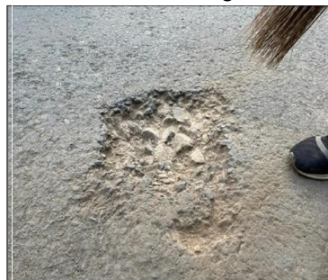
Fig- 7: Cleaning the Pothole
