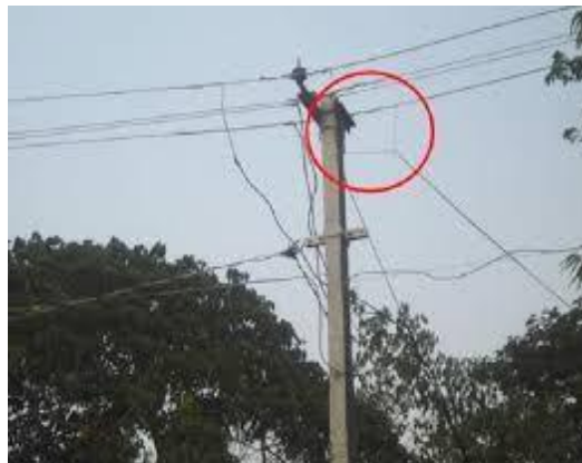
Figure 1: Tapped Transmission Line.
