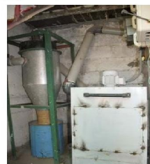
cyclone and dust collector
