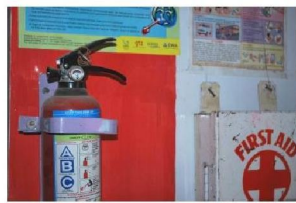
fire extinguisher and first aid kit
