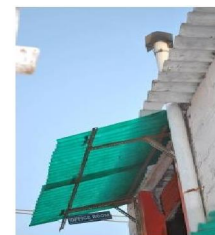
6 m high chimney
