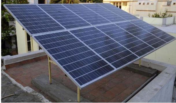
Unused area under and around solar panels
