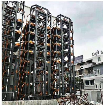
Fig 7. Rotary (Carousel) Parking System
