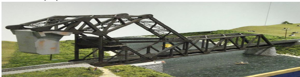
Fig. 3 Heel Trunnion Bascule Bridge
