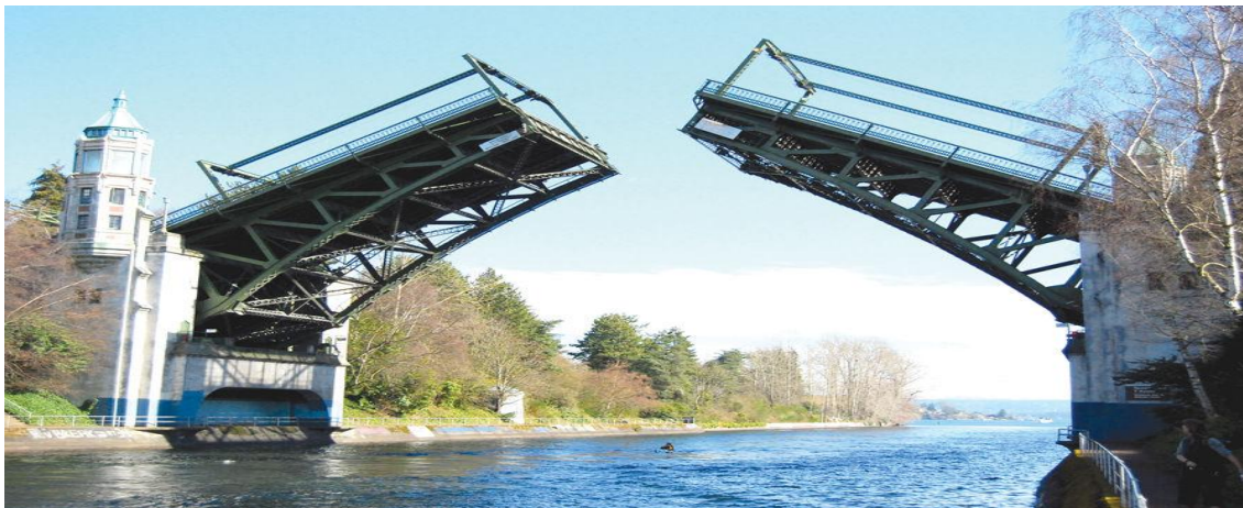
Fig. 2 Simple trunnion bascule bridge
