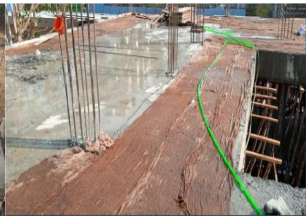
Curing of Slab
