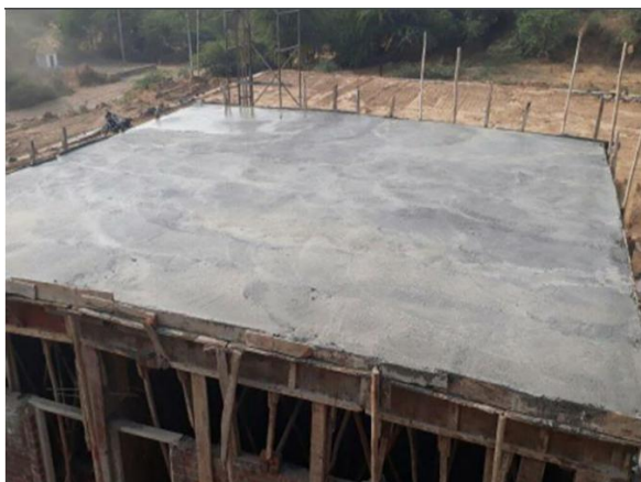
Finishing of Slab
