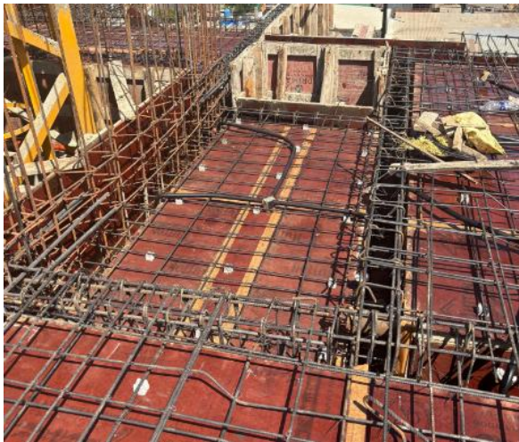
Cover provided to Reinforcement Bars Pouring of concrete using pumping method
