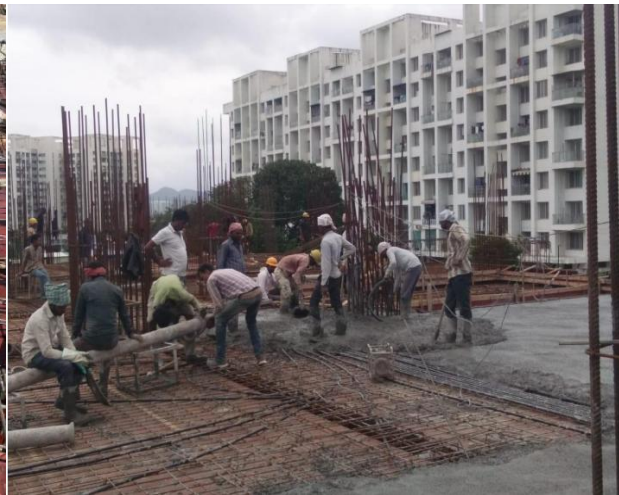
Cover provided to Reinforcement Bars Pouring of concrete using pumping method
