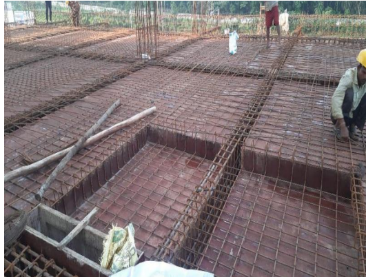
Placement of Reinforcement Bars
