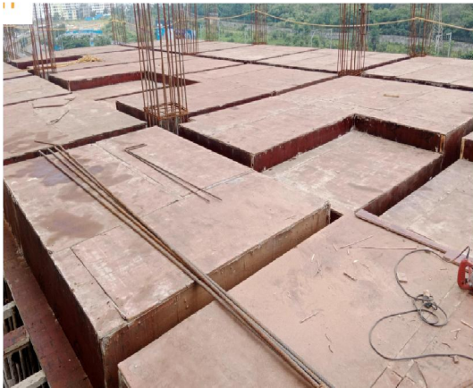
Formwork and Centering
