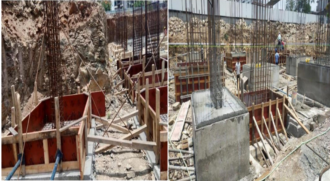
Formwork and reinforcement Isolated footings or Pad footing
