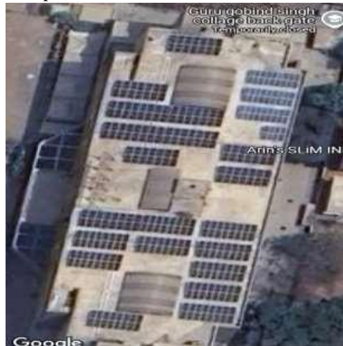
Fig. 2: GGSCOE Roof top area from Google
