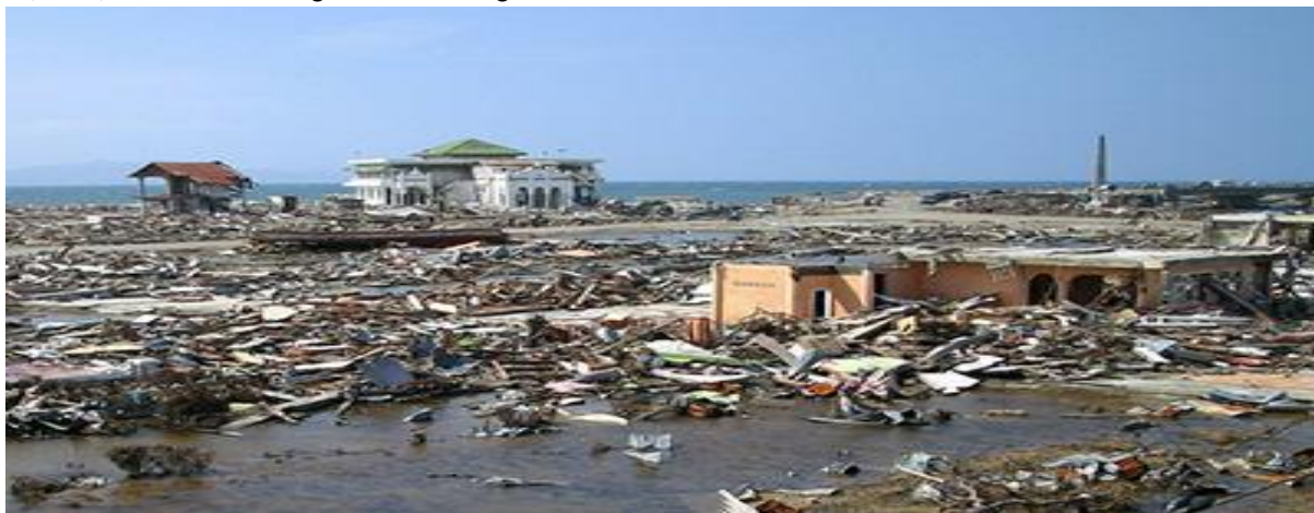
Fig.5 After Tsunami effects in India.
