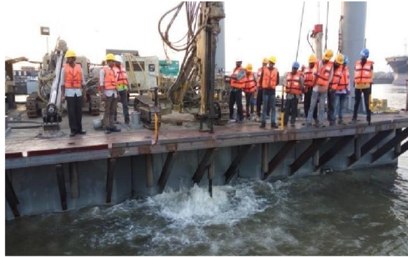
DIAPHRAGM WALL CAGE LOWERING INTO BORE HOLE
