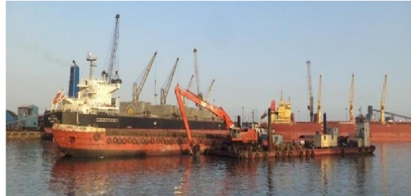
DREDGING BY EXCAVATOR
