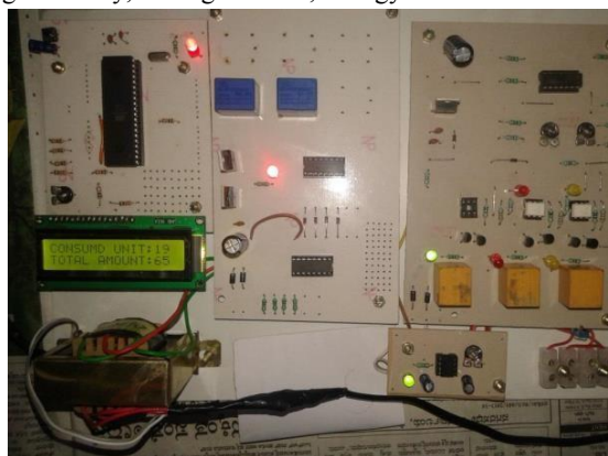
Connected Battery is Fully Charged (>5v), Energy will be Transferred to Electricity Board
