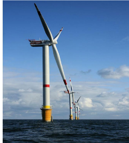
Fig. 5. Horizontal axis wind turbine
