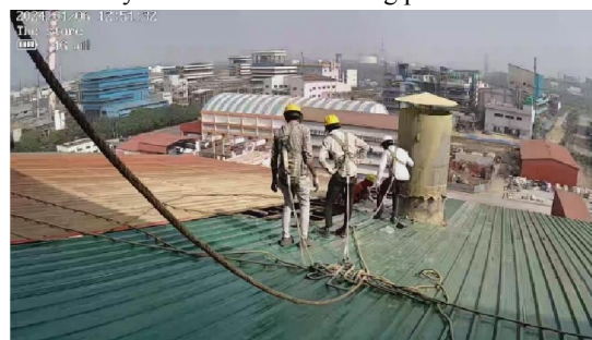
Figure 4.1: Working on Rooftop
