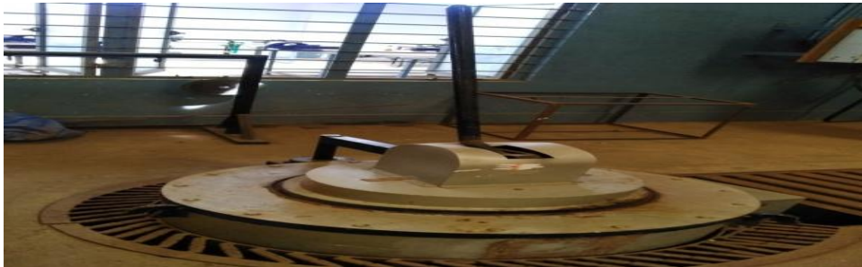
Fig. 3. Electric Pit Furnace.
