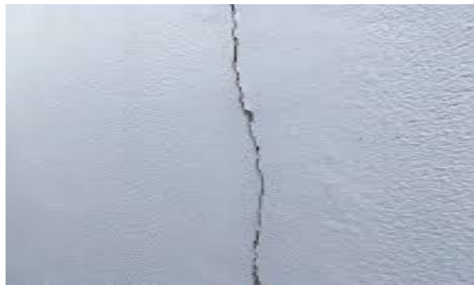
Fig.5.3 EXTENSION CRACKS
