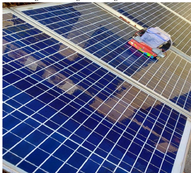
Fig. d After Cleaning of The Solar Panel
