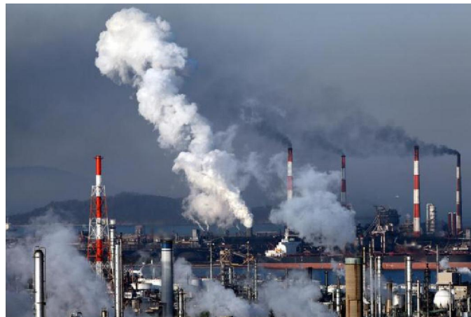
Figure - Environmental Hazard
